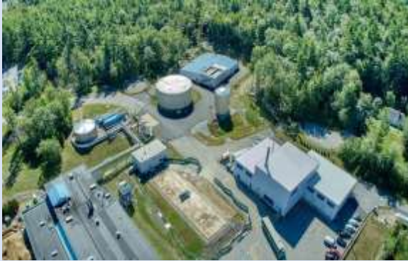
MilliporeSigma's Newly Constructed Wastewater Treatment Plant (2020). Photo: Keene Sentinel
