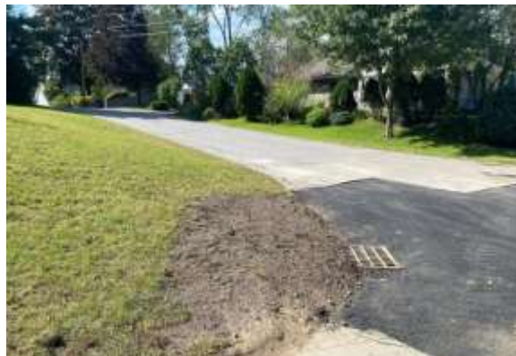
City of Keene installs catch basins to adapt to increased flooding in a neighborhood.
