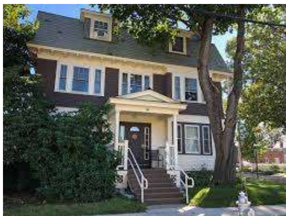
Hampshire House in Keene, now operated by Keene Housing, offers 48 rental units for people with extremely low incomes.
